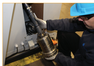
Pump* maintenance during adiabatic operation
