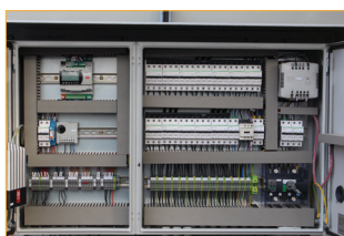
Integrated controls with separate control and power panels
