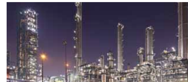
CABERO POWER PLANT COOLING
