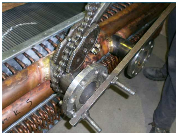
Installing screw-on flange
