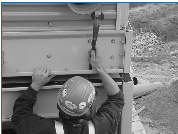
Corner alignment with drift pin
