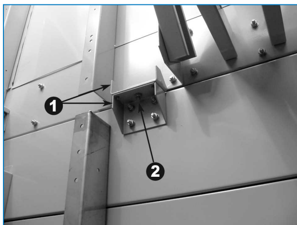
Plenum section installed on lower section
