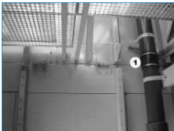
Sleeve with hose clamps
