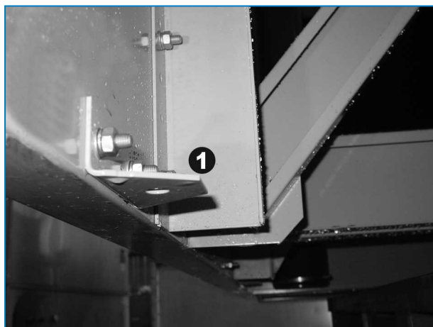
Inside view plenum section
