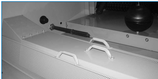
Cold water basin and basin strainer
