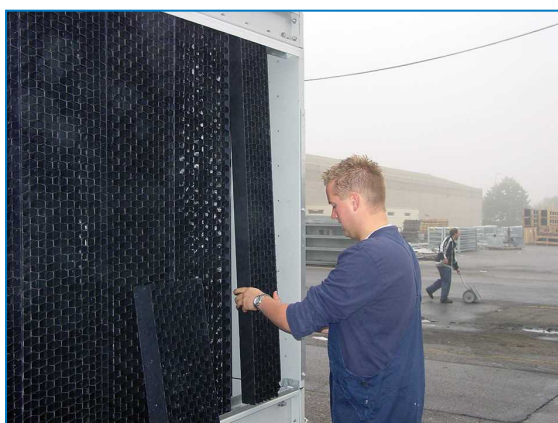
Remove combined inlet shields
