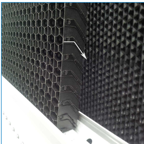
Orientation of the combined inlet shield
