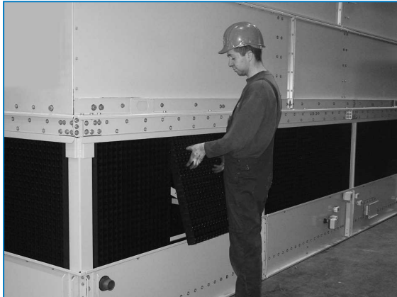
Remove combined inlet shields
