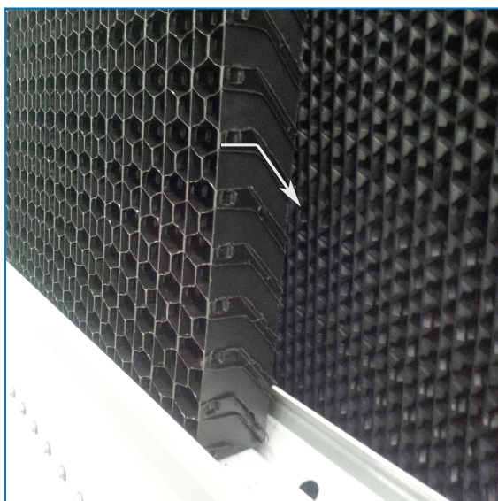
Orientation of the combined inlet shield
