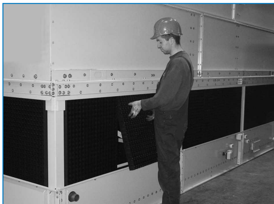
Remove combined inlet shields
