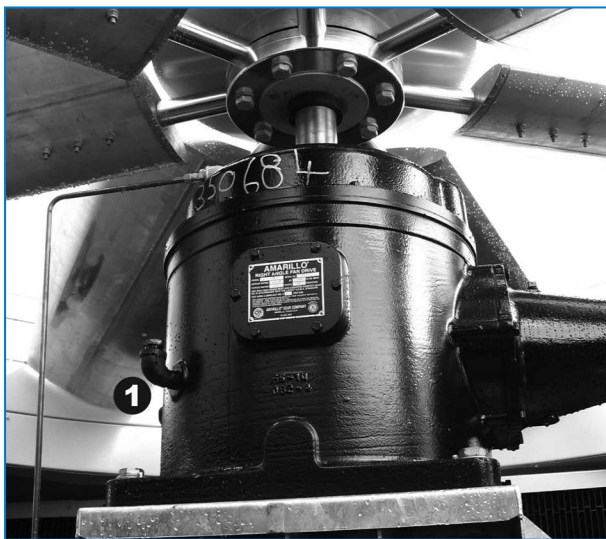
Single reduction gear drive
