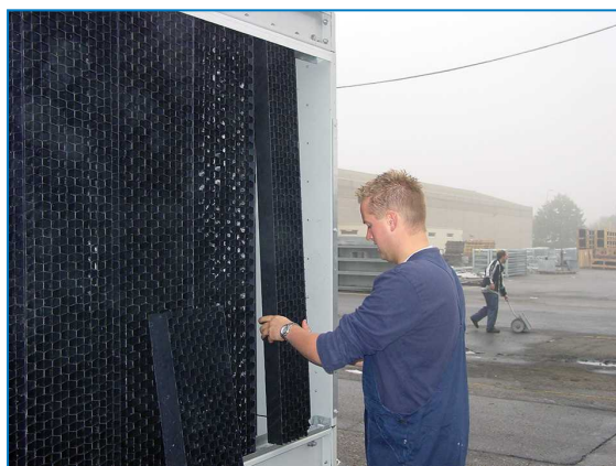
Remove combined inlet shields
