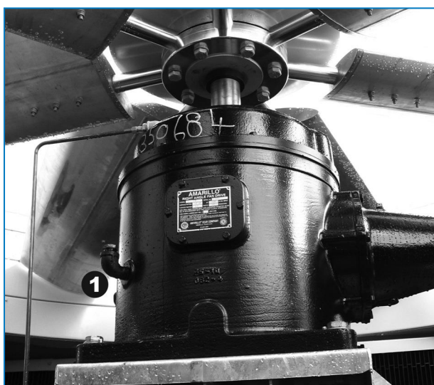
Single reduction gear drive
